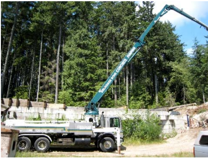
Concrete pumper ready for action.
