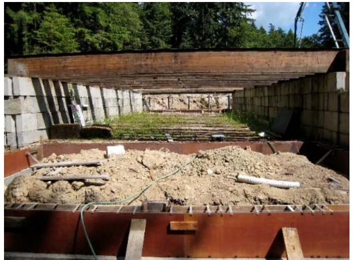
Forms ready to be filled with concrete.
